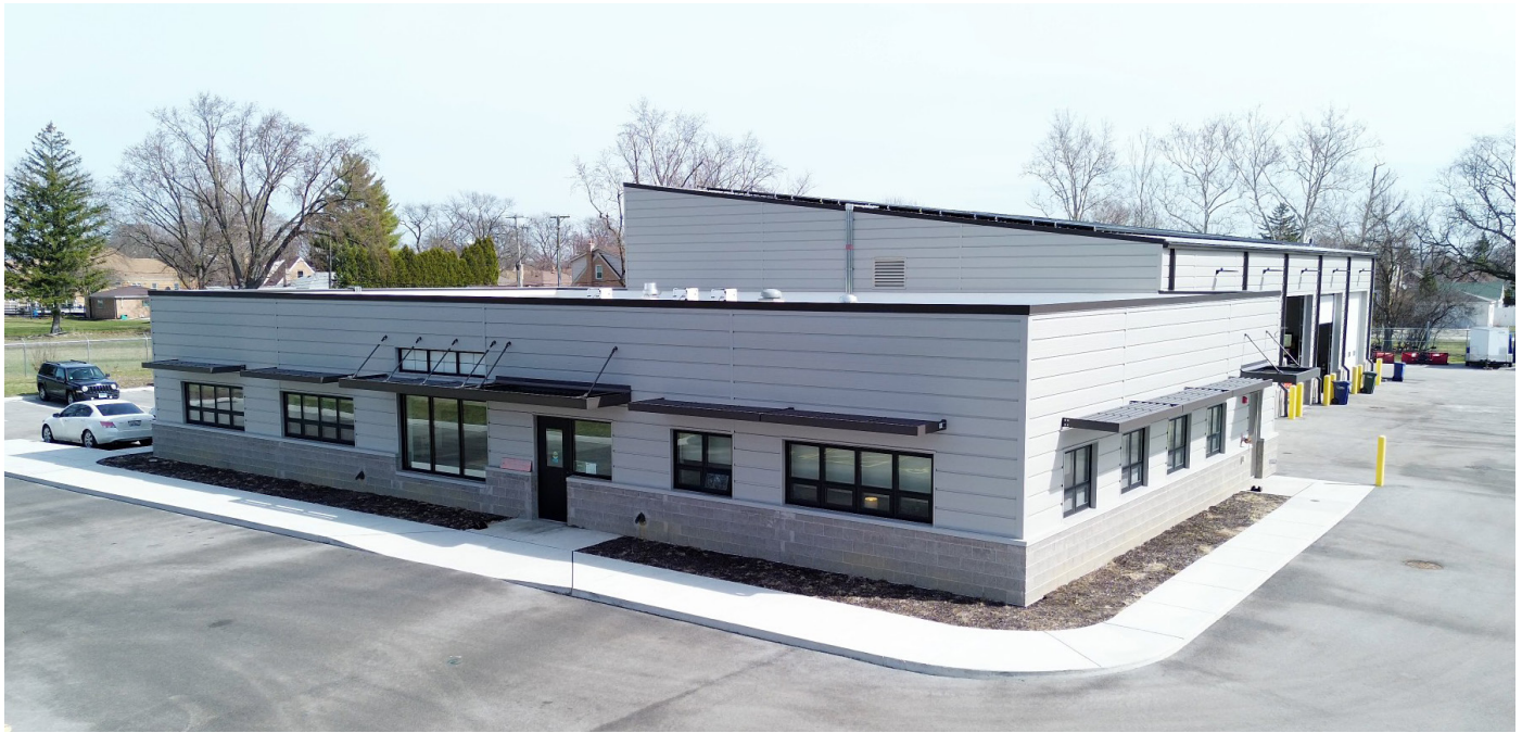
New Salt Creek Landscape Maintenance facility (photo by Forest Preserves)
