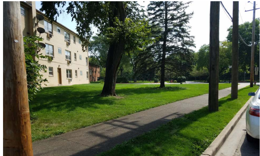
Viewing south across the property
