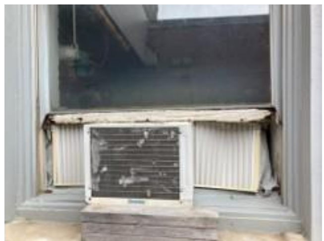
Central warehouse prior to HVAC upgrades.
